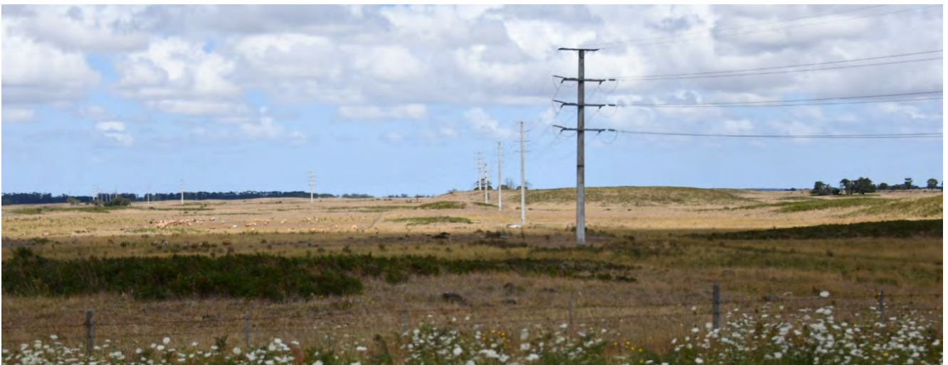
Figure 3-5 Typical medium-voltage steel monopole transmission tower
