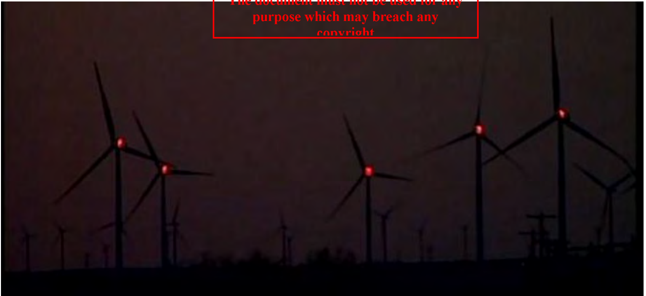
Figure 10-1 Aviation obstacle lighting example
