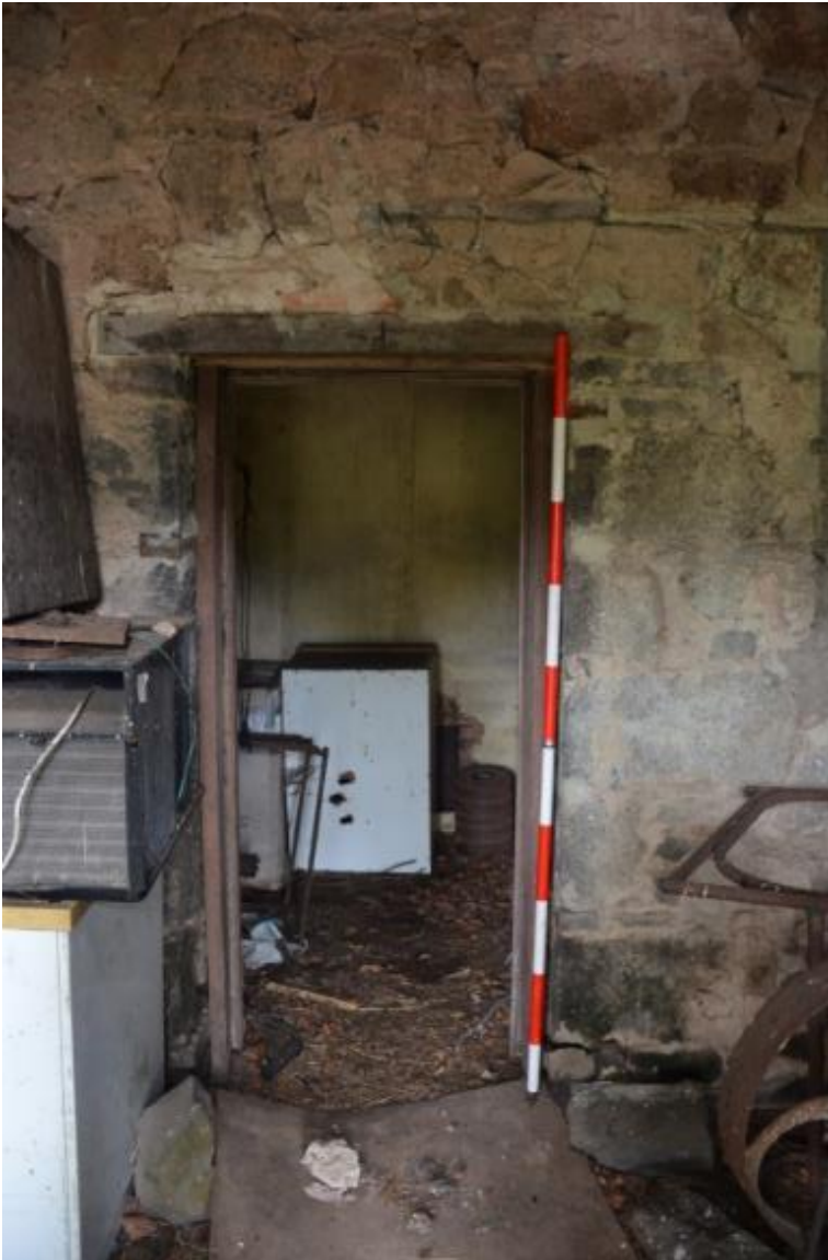
Plate 10: Internal wall showing original layout of two rooms, wooden door frame. Photo A. Wilkinson
