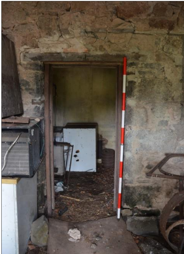
Plate 12: Internal wall showing original layout of two rooms, wooden door frame. Photo A. Wilkinson
