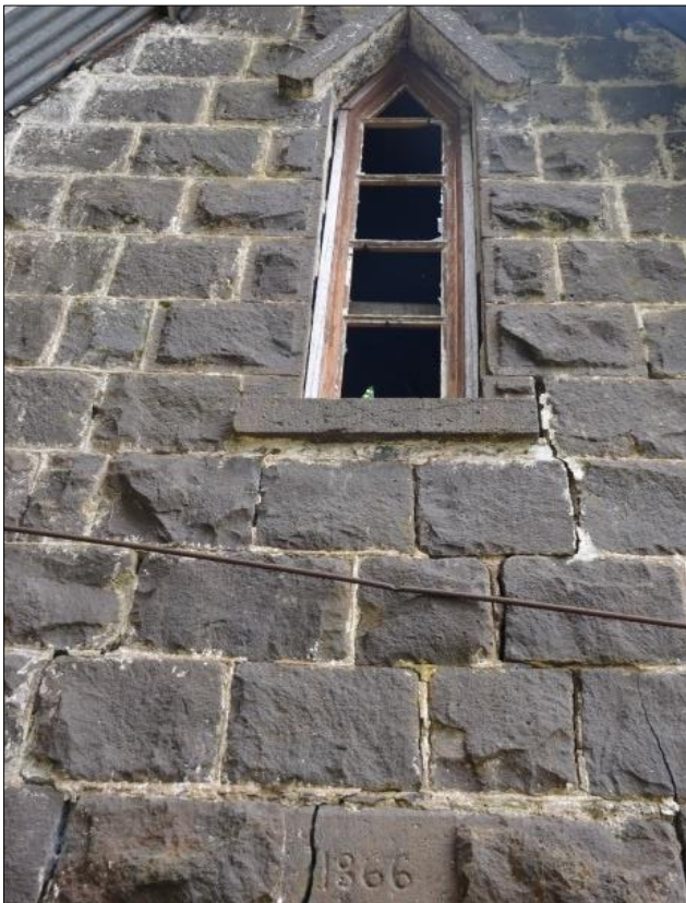
Plate 13: Detail of highlight window and stepped cracking on front of Bath House. View North. Photo A. Wilkinson
