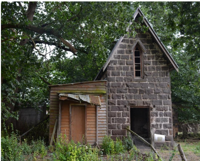
Plate 3: Dunmore Turkish Bath House, front, showing portal and highlight window and timber skillion extension built on western side, view facing north Photo: C. De Leuven
